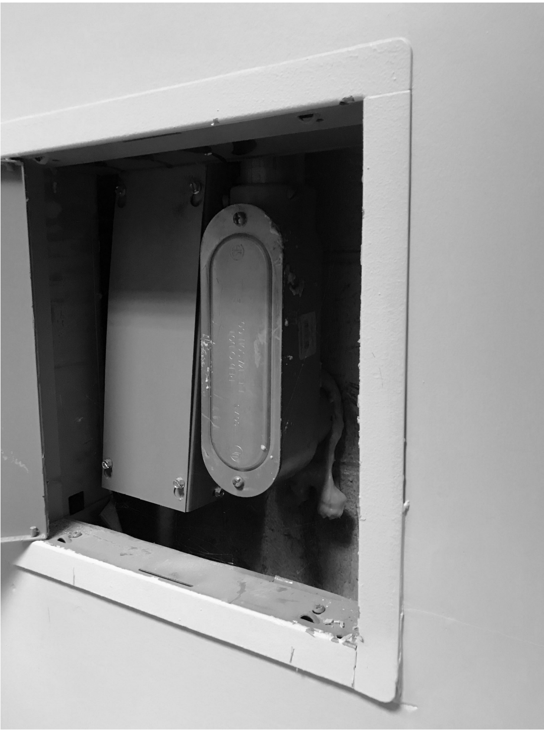
EXISTING IRRIGATION AND GARAGE LB AND WIREWAY WITHIN EXISTING HIGH SCHOOL
