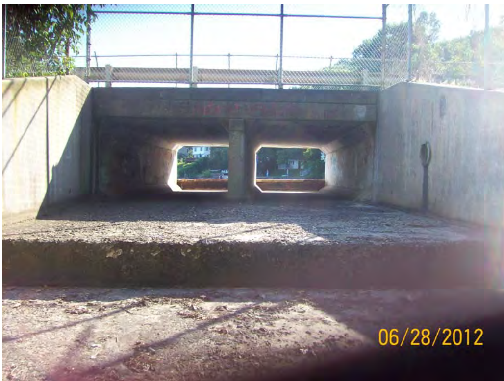
Photo 6 – Looking upstream at twin box culvert spillway. Note flashboards at upstream end
