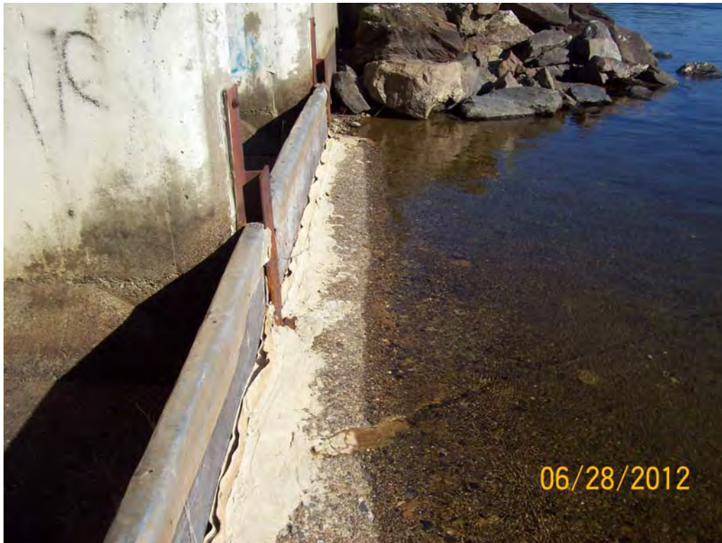
Photo 5 – Spillway flashboards and concrete approach slab.
