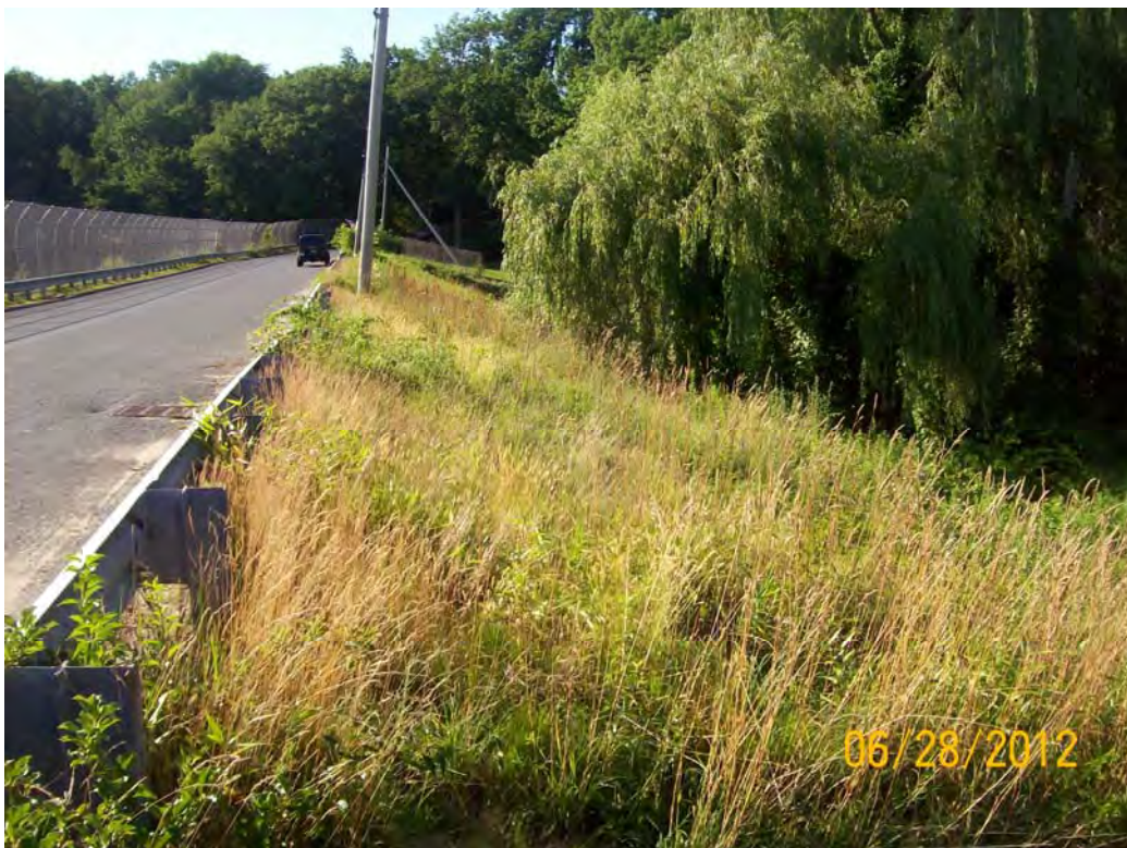
Photo 4 – Downstream slope from right abutment. Note heavy grass growth and large willow tree
