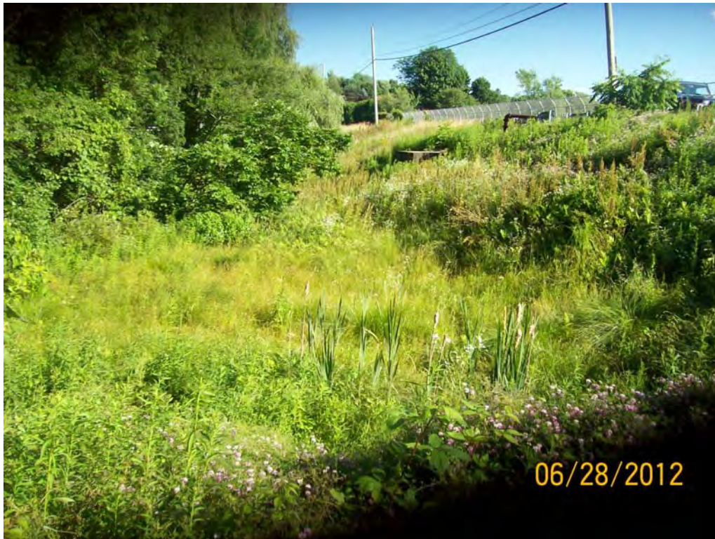
Photo 3 – Downstream slope from spillway channel. Note wetland vegetation at toe of slope due to seepage
